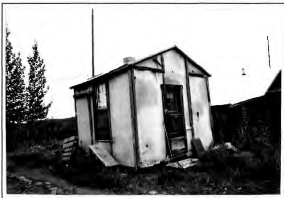
Figure 140. Bunkhouse #3, 1993. The view is looking southeast.
